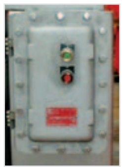
Control panel, with simple start/stop button, is suitable for remote operation
